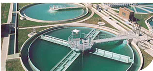
Water and waste water treatment
